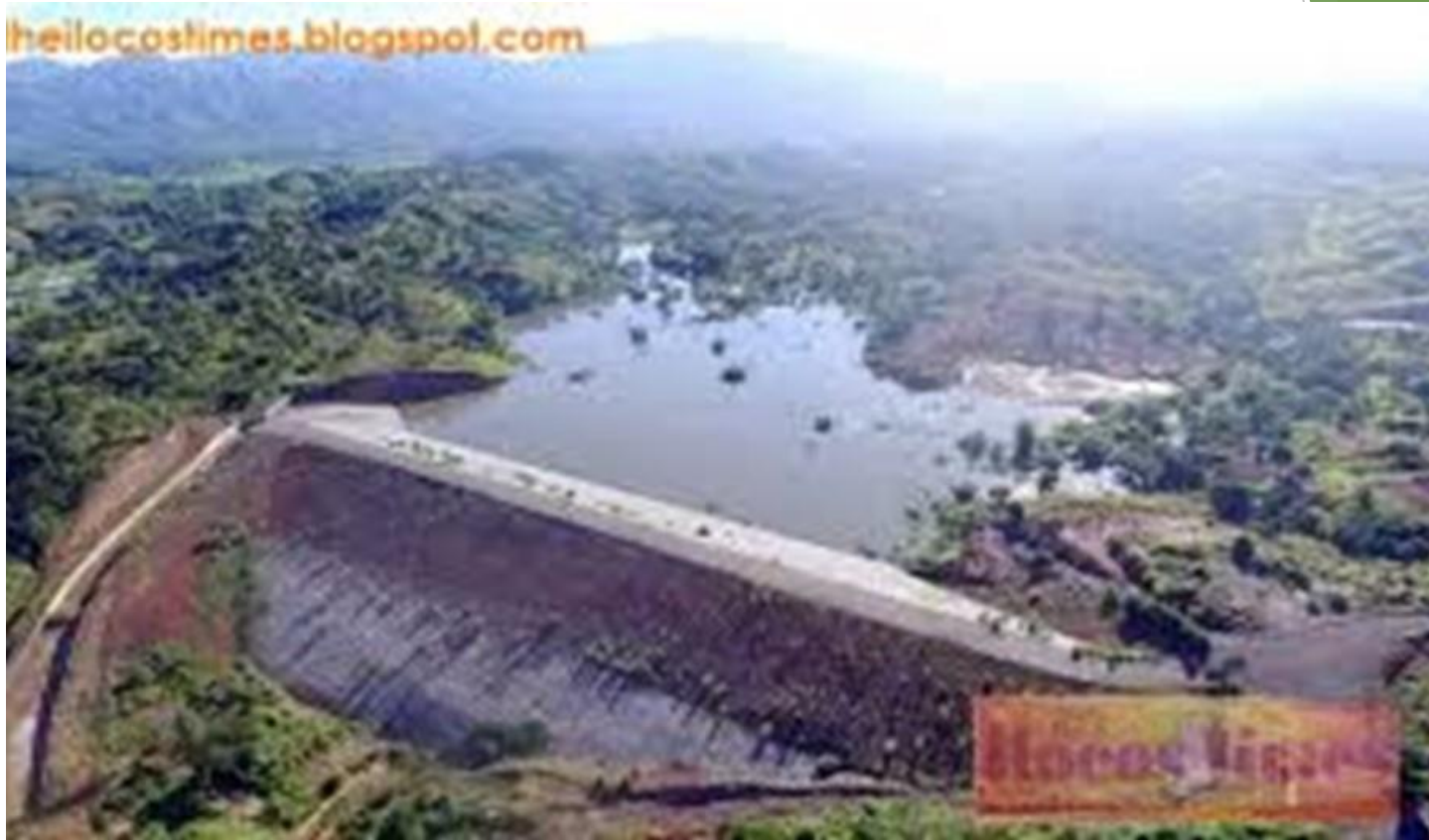
Abucay flood control cum farm reservoir with spillway
